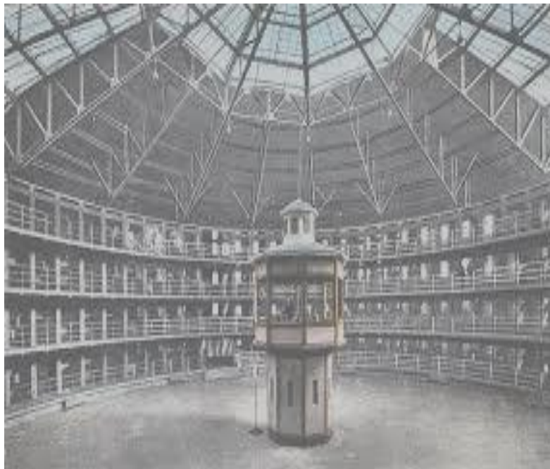
Figura 1: Stateville Correctional Center
