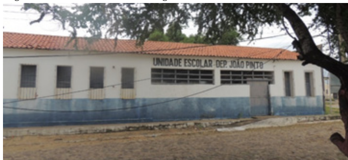
Figura 24 – Fachada Frontal Original
