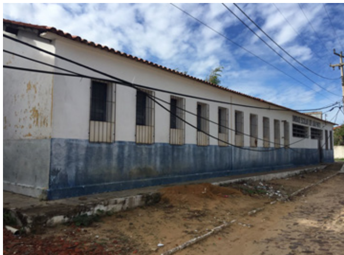
Figura 25 – Fachada Frontal Original
